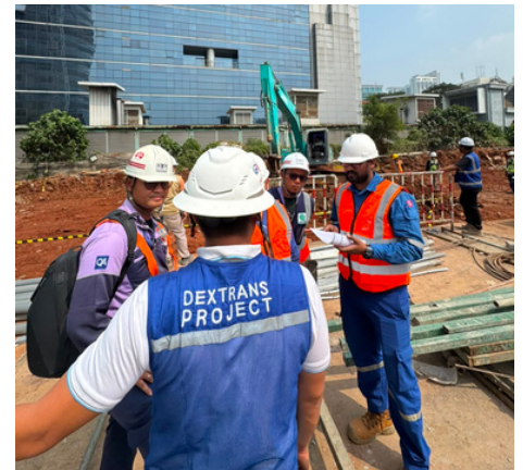
Coordinating between our Project Manager with the contractor
